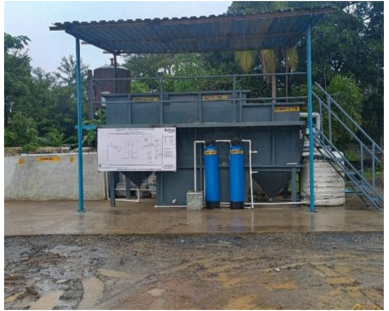
ETP of Capacity 25 KLD
